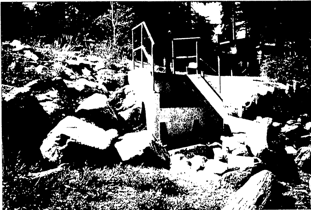
Figure 5.2. A flood control culvert empties directly into Hammond Bay, short-circuiting the lowest 220 metres of creek; fry caught in the culvert will be washed out to sea.
